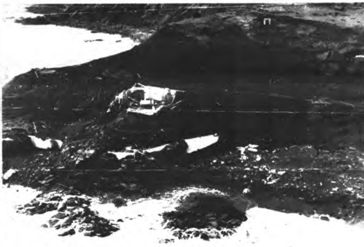
HUNDRED-FOOT "TIDAL WAVE," or tsunami, wrought impressive destruction at Scotch Cap, Alaska, in 1946. Reinforced concrete lighthouse that appears in top photograph was demolished, as shown in lower photograph, which was made from a higher angle.
